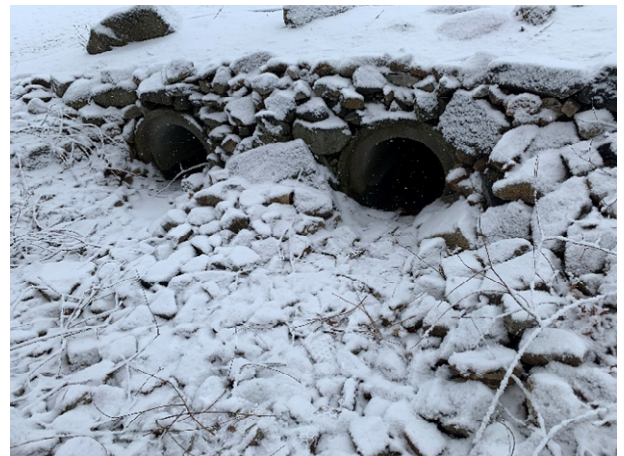
64 Gundalow - 2 (Drainage Course)
