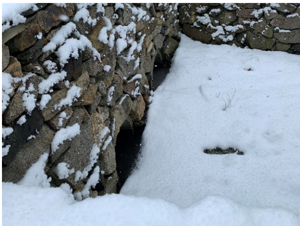
4 Brickyard Circle - 1 (Drainage Course)
