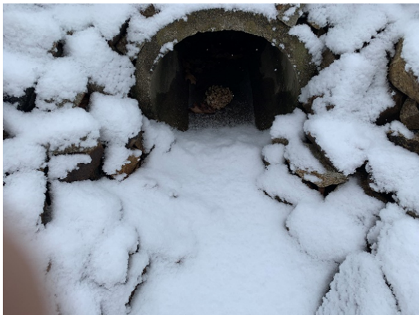
64 Gundalow - 1 (Drainage Course)
