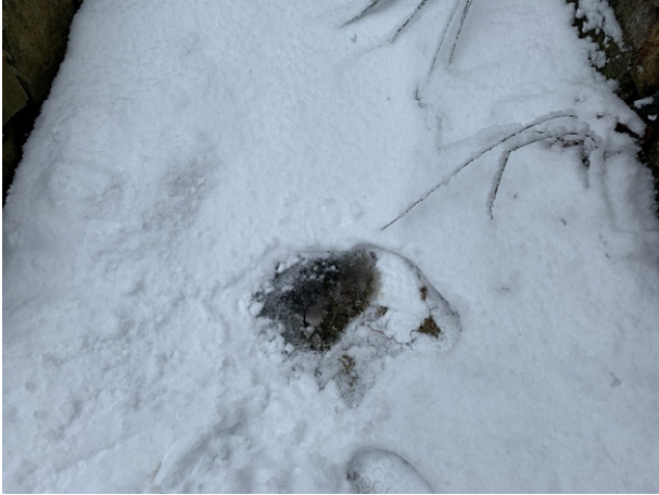
4 Brickyard Circle – 3 (Drainage Course)
