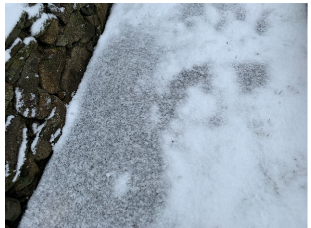
4 Brickyard Circle - 2 (Drainage Course)
